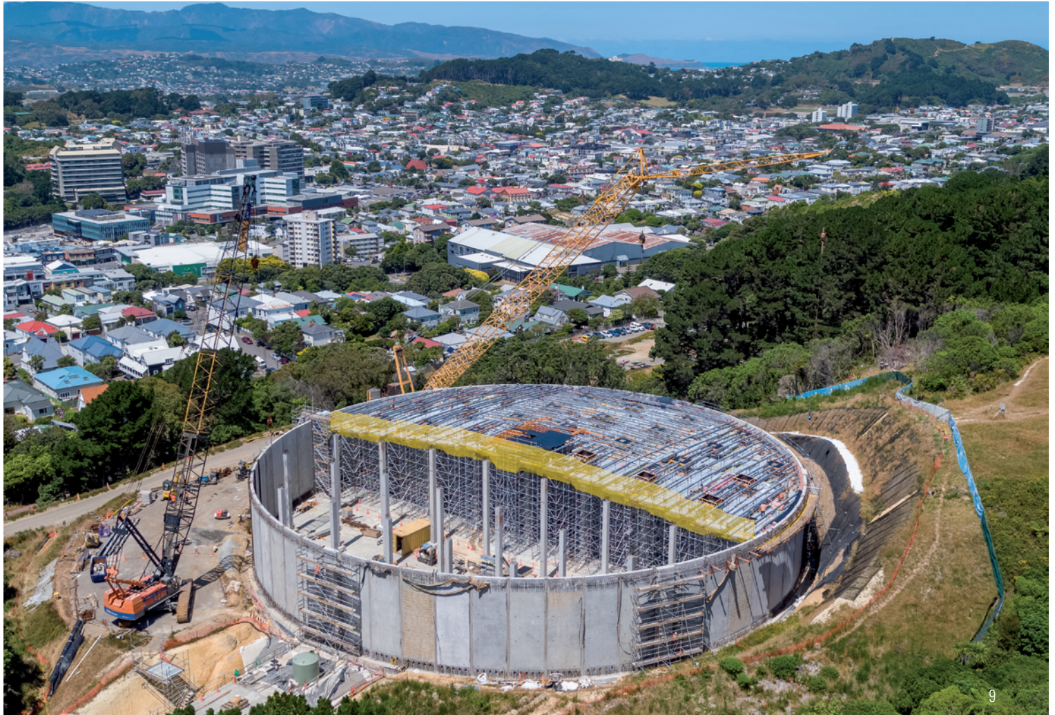
Omāroro Water Reservoir, New Zealand
