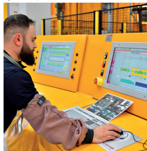
Digital control system
